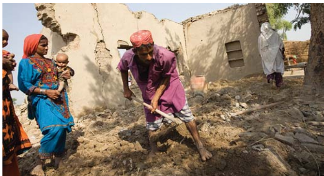
3.4 Building damage, Pakistan 📷 Marco Botelli/IOM Pakistan.
