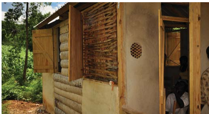
5.4 Transitional shelter materials prototype, Haiti 📷 Cordaid Haiti.
